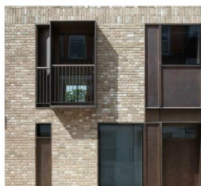
BB STEEL BALUSTRADE Flat solid pane vertical steel tube balustrade Colour to match AF/G
