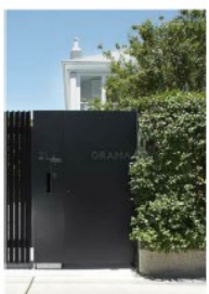
FC11 FENCE TYPE 1 Metal framed vertical steel fence - painted black FC12 FENCE TYPE 2 Solid metal gate FC13 FENCE TYPE 3 Square end capped timber fence - 1.5m - 1.8m high Cladding fence between apartments of rear Floor boundary fence Colour to future selection
