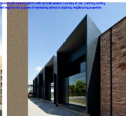
PF7 METAL FINISH TYPE 3-METAL HOODS Curved, Metal Champagne Bronze or similar
