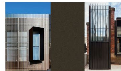
PF17 METAL FINISH TYPE 4 Project metal facade windows Metal panel cladding Colour powdercoat modern/black bronze colour generally
